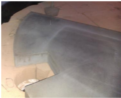
Preparation of insulating hole and arrange the prepared segment
