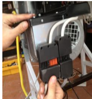
Connect the multi-polar connectors of the switchgear and the valve group to the burner
